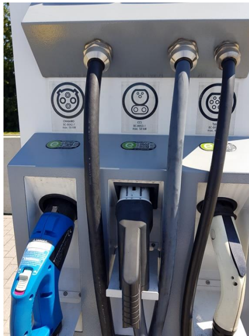
Figure 6: Multi-standard charger (CHAdeMO, CCS, Type 2) funded by the CEF 16
