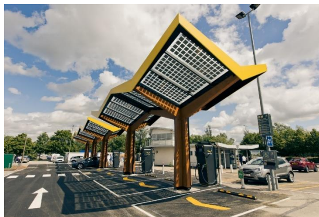
Figure 16: A charging hub with a photovoltaic roof 29
