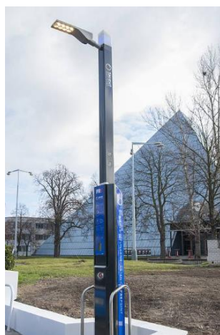
Figure 19: A street light combined with an AC charging station 32
