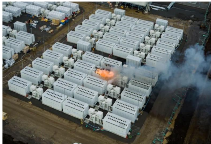
Figure 12. A fire in a 13-ton shipping container of Li-ion batteries in the Tesla Megapack battery storage facility in Australia 32
