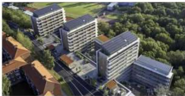
2 nd life Bus batteries and battery system used in the apartment complex in Gothenburg. Source: Ylva Olofsson's presentation
